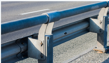
Installing barriers to keep people out of the way of vehicles
