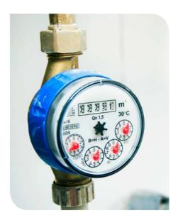
or black on a white background. Now read the dials that are red and white. These indicate how many litres of water you have used. The red and white dials will move quickly when water is being used. There are normally three or four of these dials, although sometimes the fourth one is located separately on the meter face (it indicates how many tenths of a litre you use).
