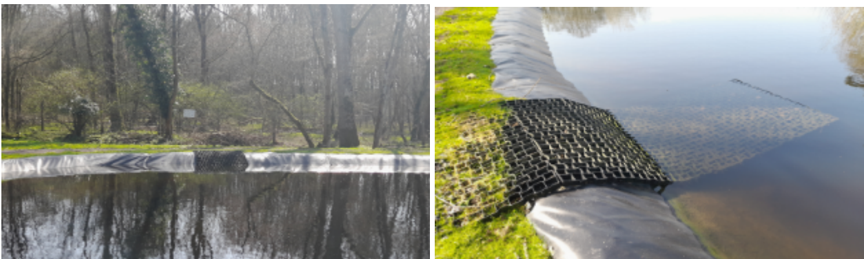
Figure 2 (left) and Figure 3 (right): showing the installed netting ladder within Lagoon One at Tidworth STW.
