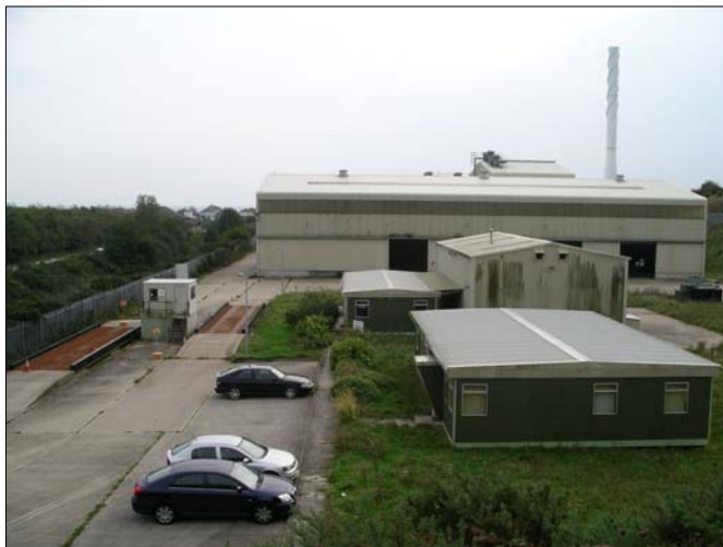
Figure 2.1 Application site viewed from north
